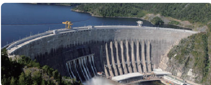
Water Conservancy Monitoring
