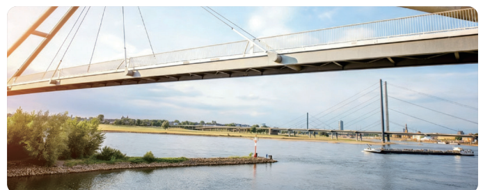
Transportation Infrastructure Monitoring
